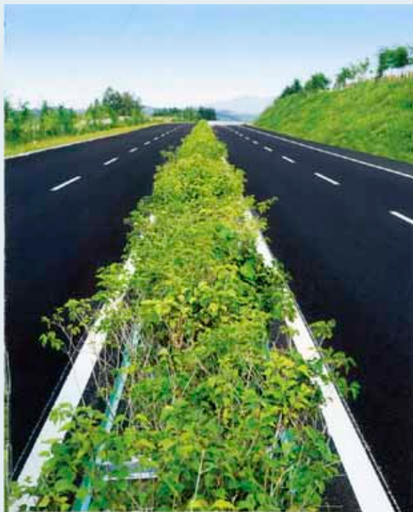
Figure 2. Shrub median between connected guardrails on a new expressway. From Big Spanning by Sheng TaiLu et al., eds. 2008. Jilin Provincial High Class Highway Construction Bureau, Changchun, China.
