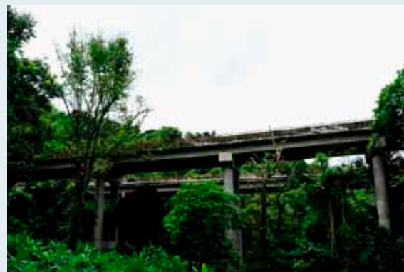
Figure 6. Highway across valley to facilitate the movement of floodwater and wildlife. Copyright Marcel Huijser.
