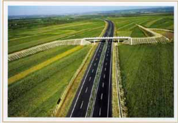
Figure 4. New expressway built on farmland showing narrow median, shoulder and roadside, plus characteristic erosion-control structures on fill-slopes. From Big Spanning by Sheng TaiLu et al., eds. 2008. Jilin Provincial High Class Highway Construction Bureau, Changchun, China.
